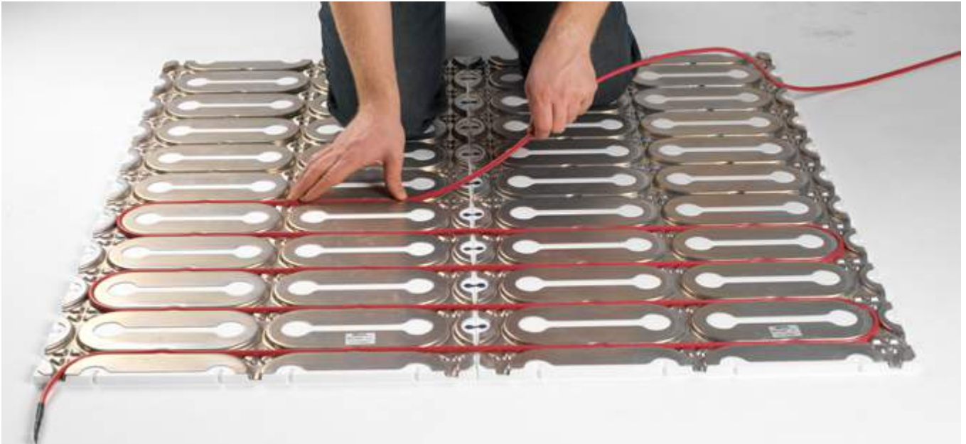
Fig. 20. Mounting method for heating cable into Reflect insulated plates (EFCI Dry)
